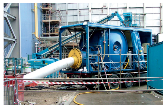
CIPP installation unit
