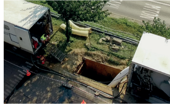
Liner installation with inversion system
