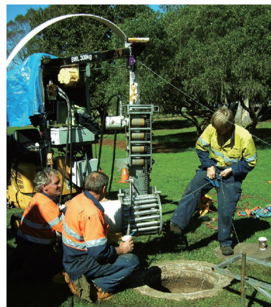
Manhole Installation.
