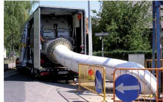
CIPP installation unit
