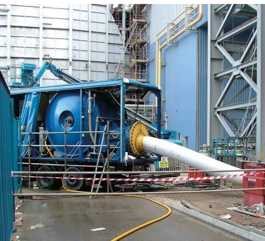
TUBETEX – the optimal solution for trenchless pipe rehabilitation of pressure and industrial pipes
