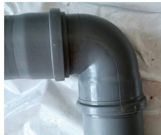
The flexible fabric allows for the rehabilitation of 90-degree-bends
