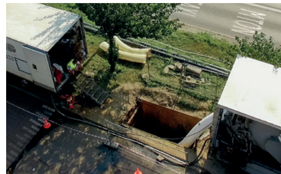
Liner installation with inversion system
